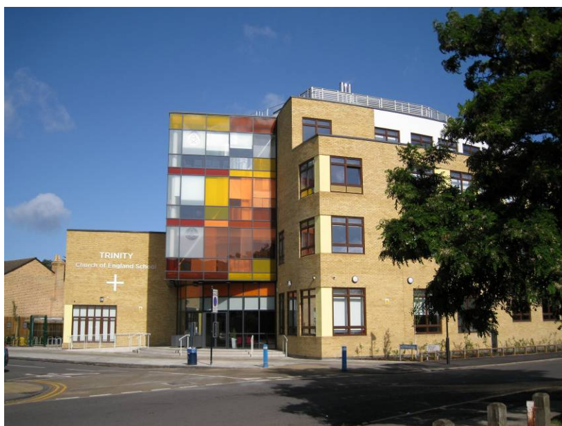
Main entrance showing the distinct coloured glass
