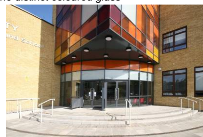
Entrance beneath building cantilever
